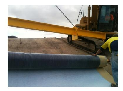
unrolled down the dam face using a backhoe and spreader bar assembly. It is important to seal the overlaps with bentonite clay. Finally 30cm of cover soil is placed over the GCL. Once laid, vehicular traffic should be avoided.
